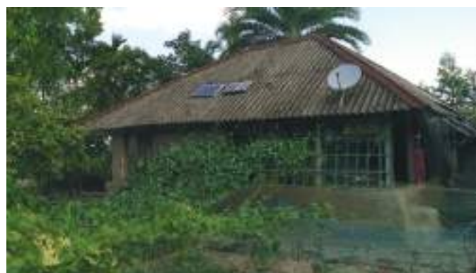
Image 3: Autonomous adaptation – solar energy and raised floor height
